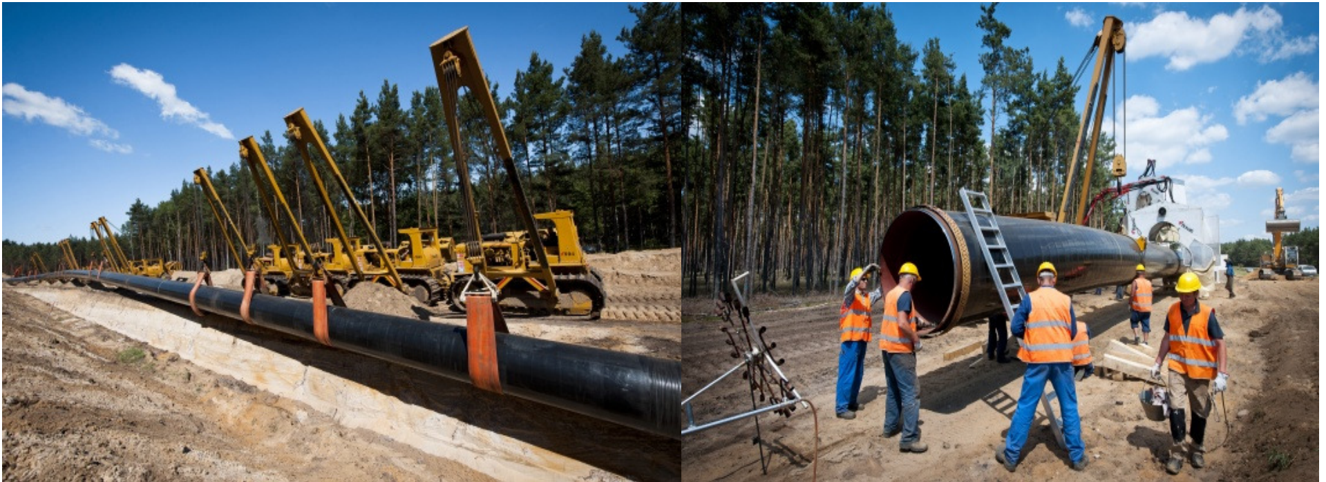
OPAL PIPELINE PROJECT
