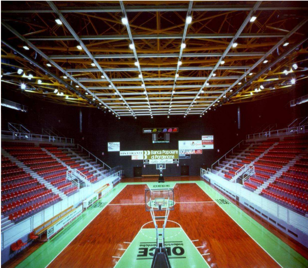
Structure: New sports hall - roof structures involving primary & secondary trusses from hot rolled sections.
